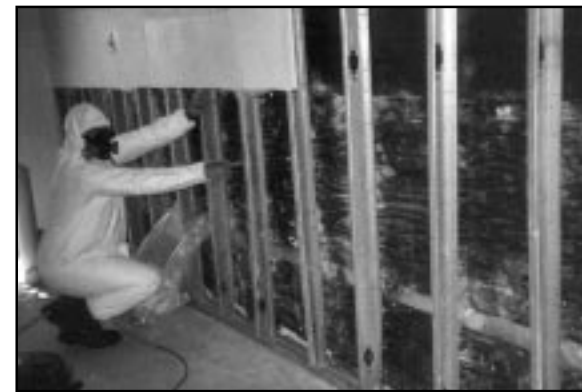
Worker remediating mould from a leaky building.
